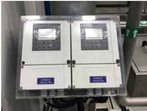
喷嘴堵塞实时监测功能 Injection Nozzle Block Or Not Real Time Monitoring
